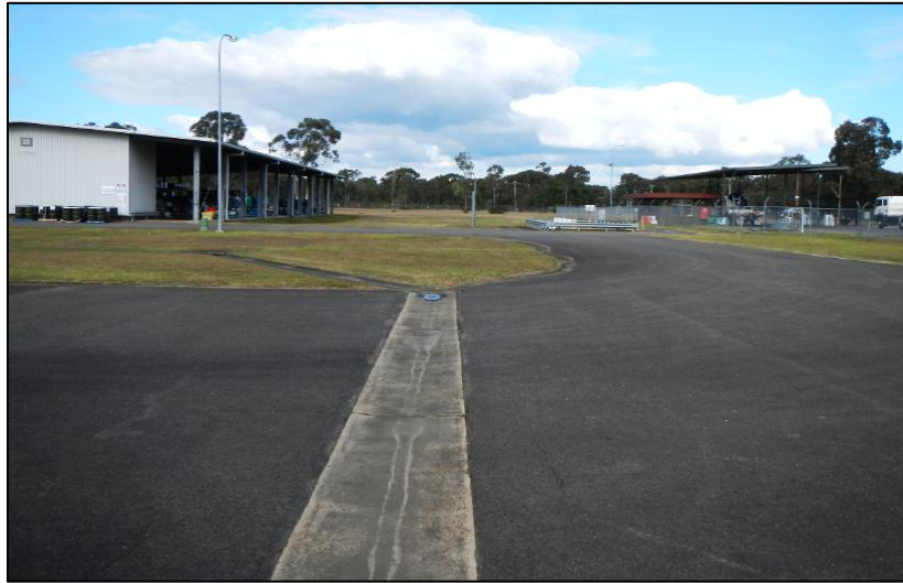
Figure 29: Southern portion of Stage 1A area, facing south.
