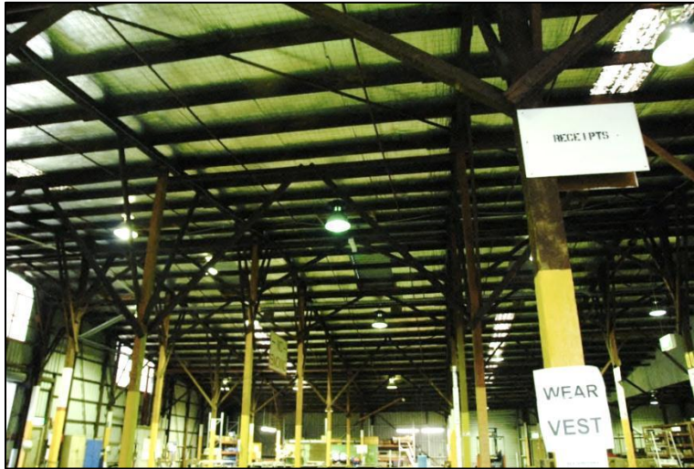
Figure 16: Interior of Building 75, showing original timber post and beam construction
