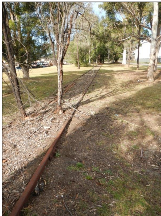
Figure 17: Railway line opposite Buildings 17 and 18
