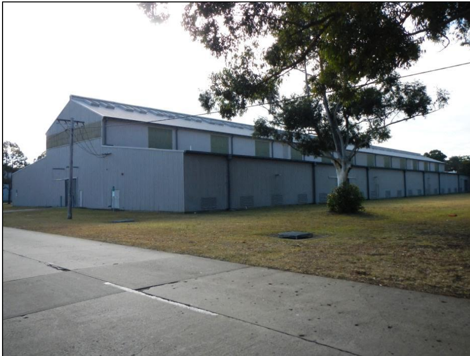
Figure 14: Building 7, at the centre of the DNSDC - a typical WWII composite timber and steel crane-served warehouse building
